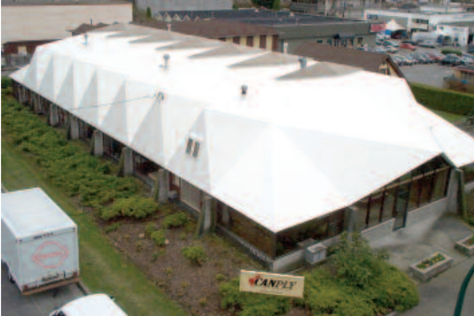
An aerial photograph of the Canadian Plywood Association head office and technical centre. The building was officially opened in 1962 and is still pleasing to the eye over 40 years later! Its dramatic roof line is faceted with 86 triangular and trapezoidal panels of plywood.
